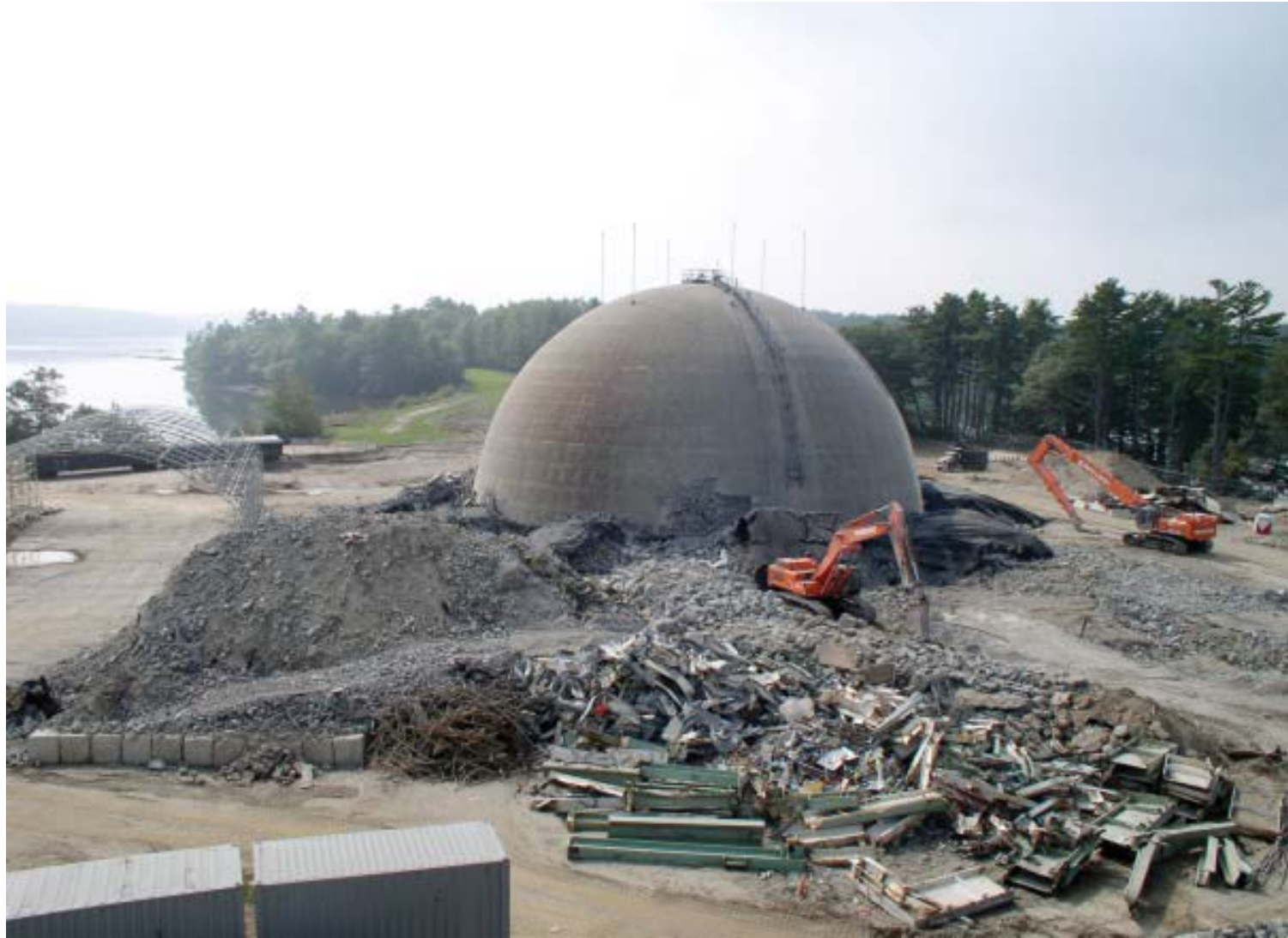
Containment following explosive demo
