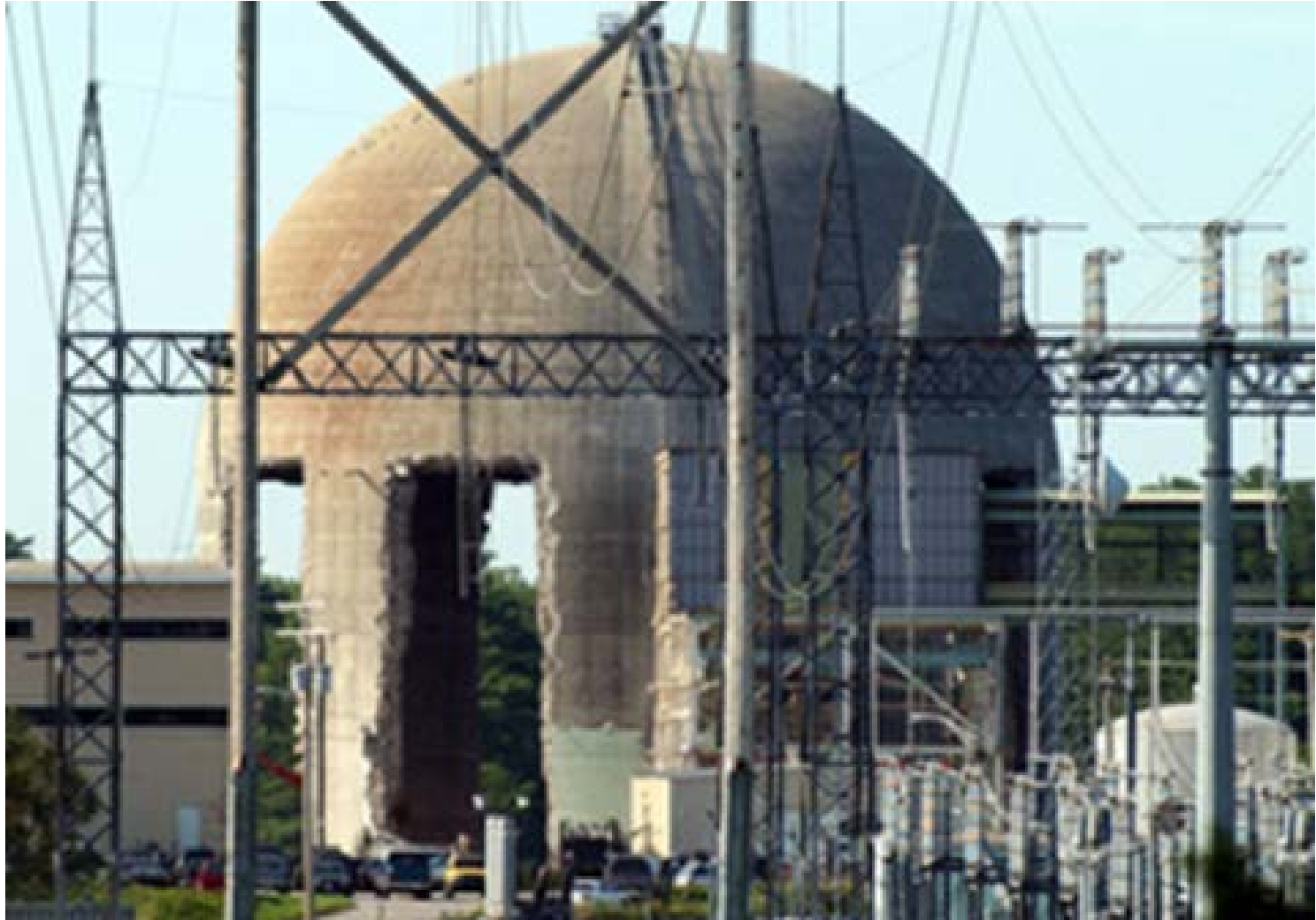
Containment being prepared for demolition
