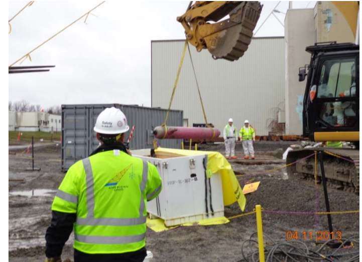
Waste Characterized, Segregated and Packaged Throughout Demolition
