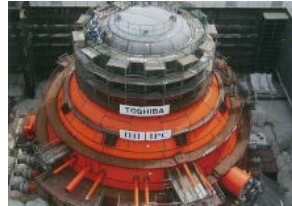
Containment Vessel (PCV)
