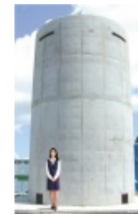
Spent Fuel Storage Facility
