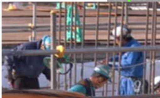
Workers in the G zone
