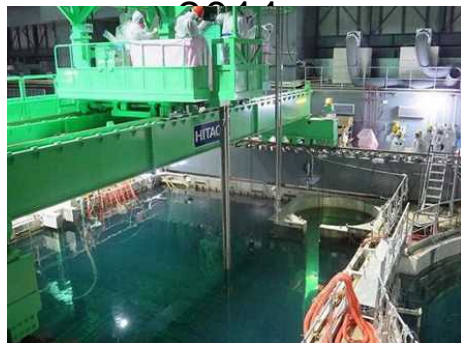
Process of removing fuel rods at SFP Unit 4
