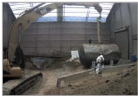
2011: Removal of Tank W1A at ORNL
