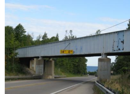
Low Overhead Bridge Near Big Rock Point
