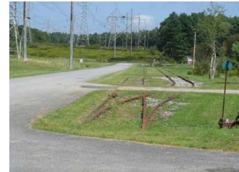
Current Condition of Onsite Rails at Maine Yankee
