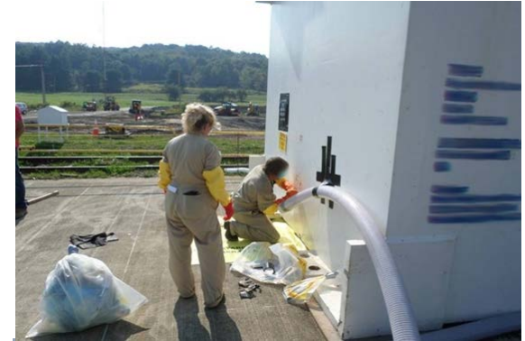
Melter Grouting Operations
