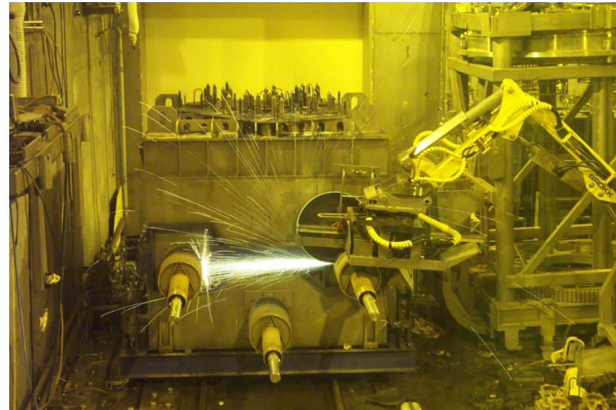
Preparing the Melter for Removal and Packaging
