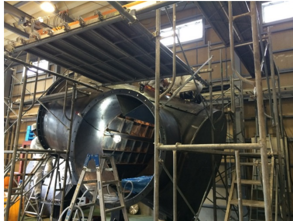
Figure 5 – Full scale mock-up with V-gap insert installed.
