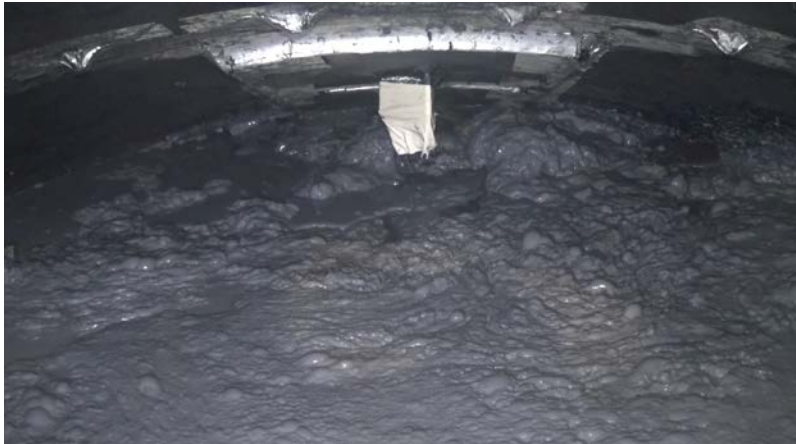
Figure 17 - U-gap plug as seen from gap entrance.
