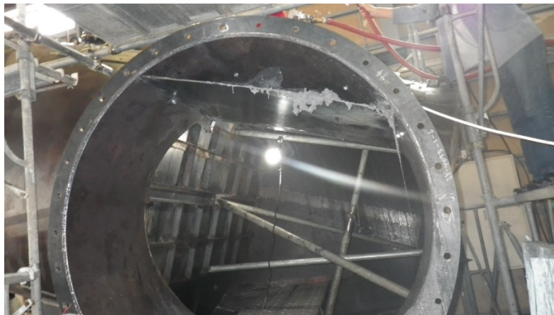
Figure 16 - U-gap plug as seen from branch.
