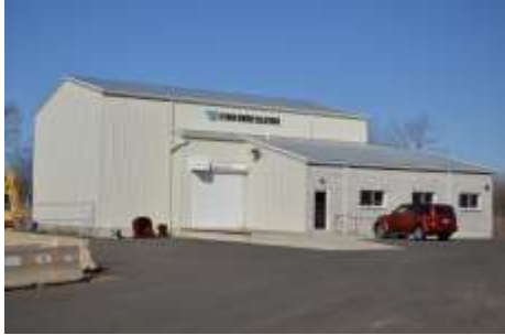
Figure 1 – VJT High Energy facility located at East Haven Connecticut.
