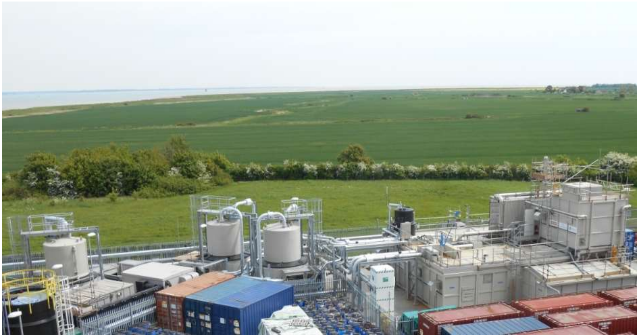
Figure 1. ADAP plant at Bradwell power plant, UK
