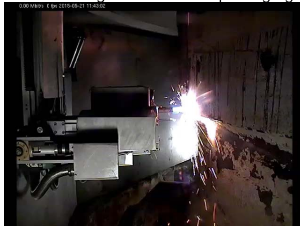
Fig. 5: Remote controlled thermal cutting segmentation of RV
