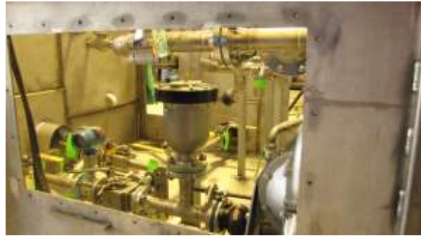
Fig. 8: Transfer Line Service Box (being fabricated)
