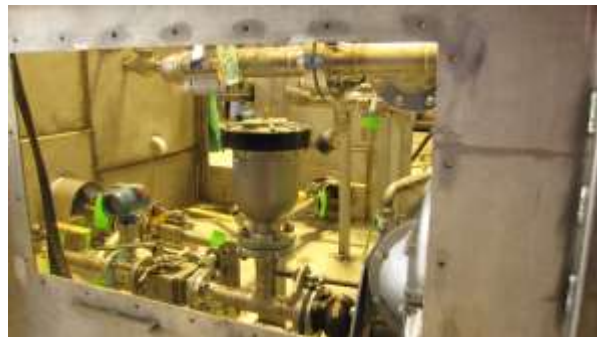
Figure 8: Transfer Line Service Box (being fabricated)
