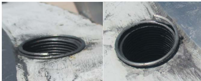
Figure 1: Heli-Coil Threaded Insert backed out from closure bolt hole on 8-120B cask
