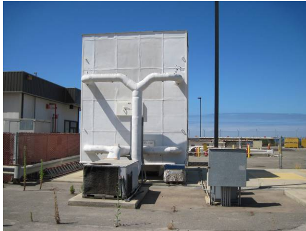
Figure 1 RCP #2 located in South Yard
