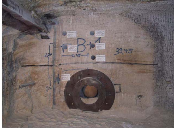
Figure 5. Photograph of the BAMBUS II re-excavation.
