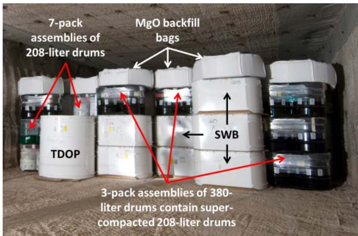
Fig. 2. Typical payload containers emplaced in a disposal room underground at WIPP, showing a nominal payload container type mix.
