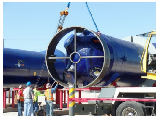
Figure 7 A/B – Impact Limiter Rigging
