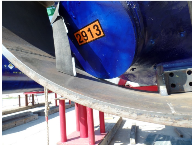
Figure 8 – Tight Fit Up
