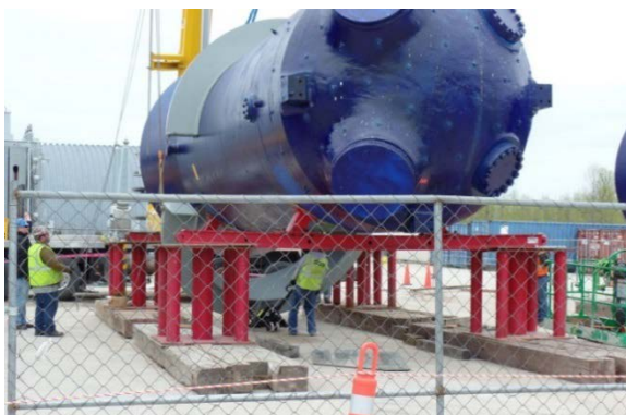
Figure 7 A/B – Impact Limiter Rigging
