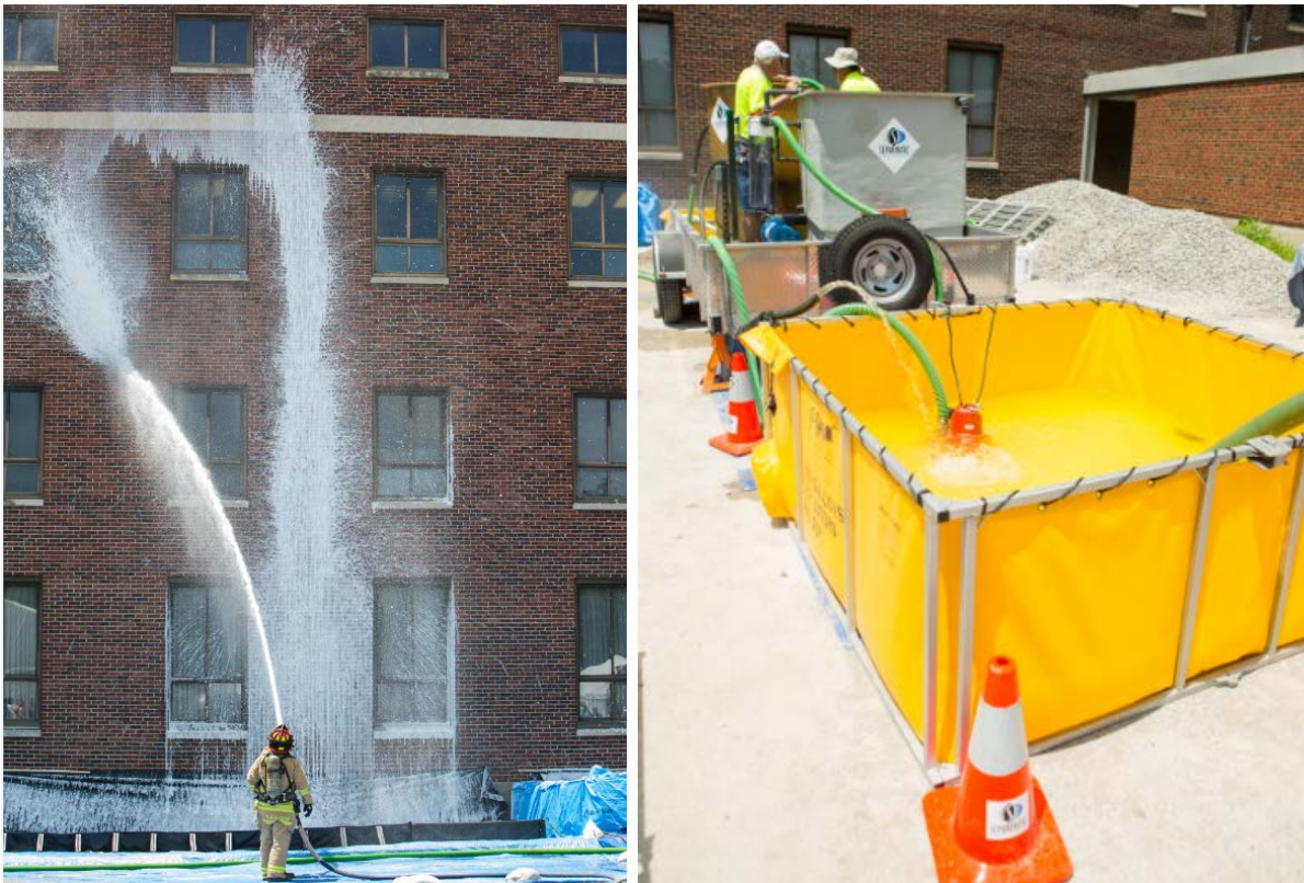
Figure 5. Application of Environment Canada foam via a fire truck (left). Water reuse system of IWATERS (right).
