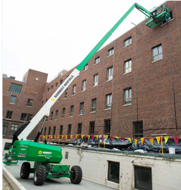
Figure 3. 20 m-boom lift that was used to safely reach the higher elevations during the scalability demonstrations.
