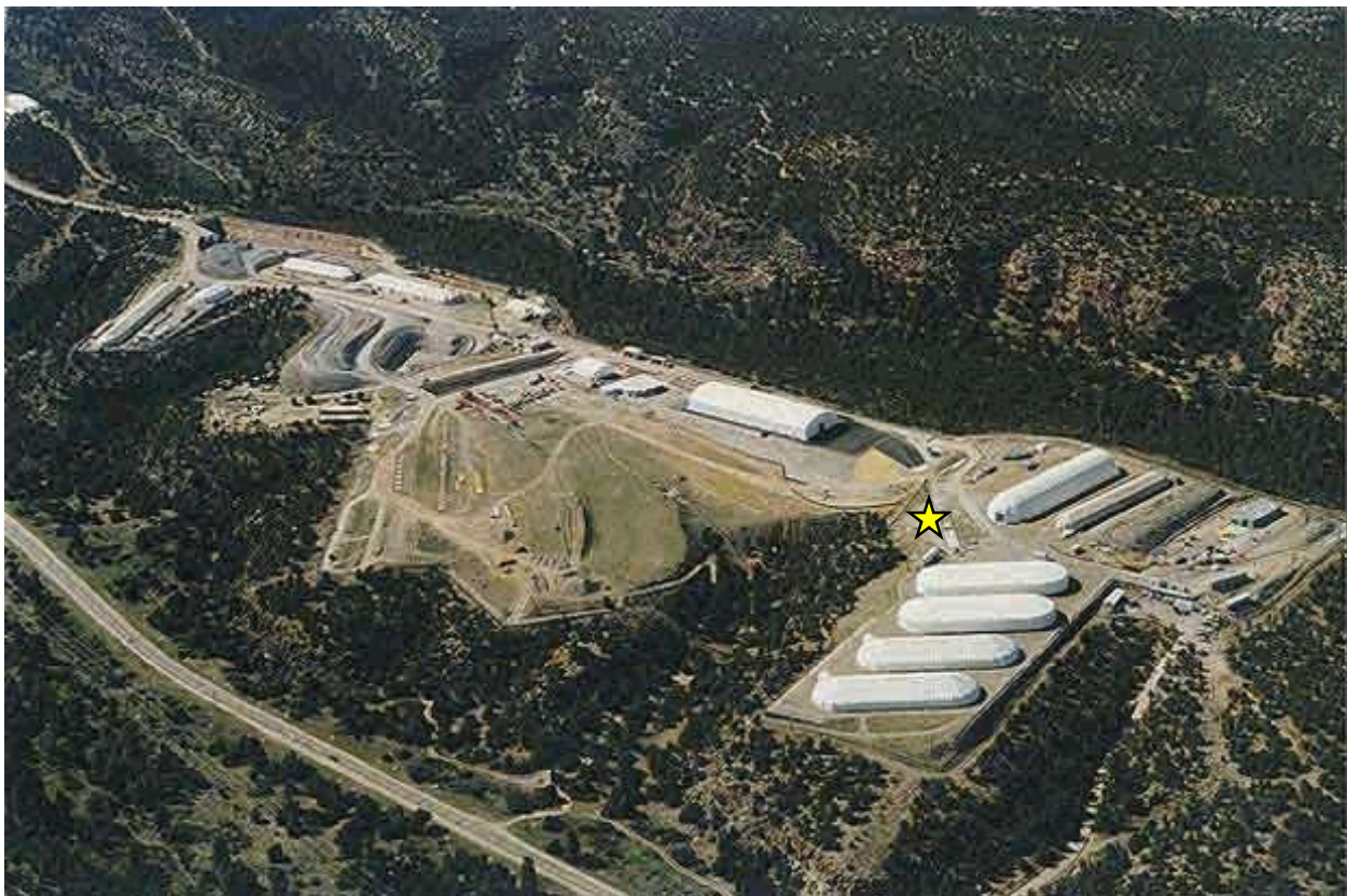
Figure 2: Location of remote handled TRU shafts are MDA G, Los Alamos National Laboratory
