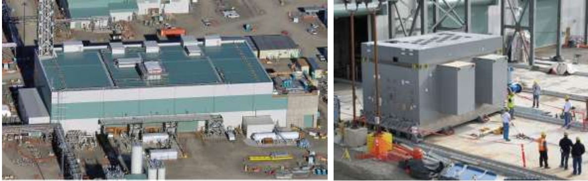
Figure 6 – WTP Low-Activity Waste (LAW) Facility and Melter
