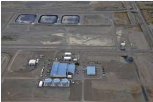
Figure 12 – Liquid Effluent Retention Facility (LERF) and Effluent Treatment Facility (ETF)
