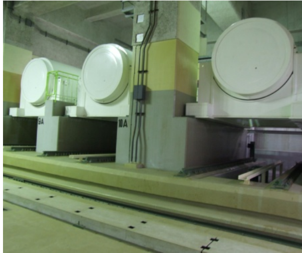
Fig. 7. TN-24 Storage casks stored at Fukushima in Japan.
