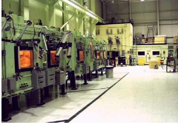
Fig. 4. IFTF Warm Cells before decommissioning
