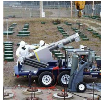
Fig. 3. Test lift to retrieve degraded fuel
