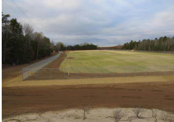
Fig. 11. Legacy waste burial area with cover installed
