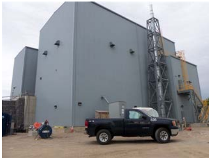
Fig. 1. FPS facility at CRL
