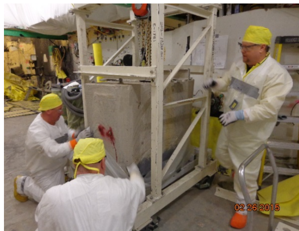
Figure 5. A concrete hatch block is transported on the lifting frame.
