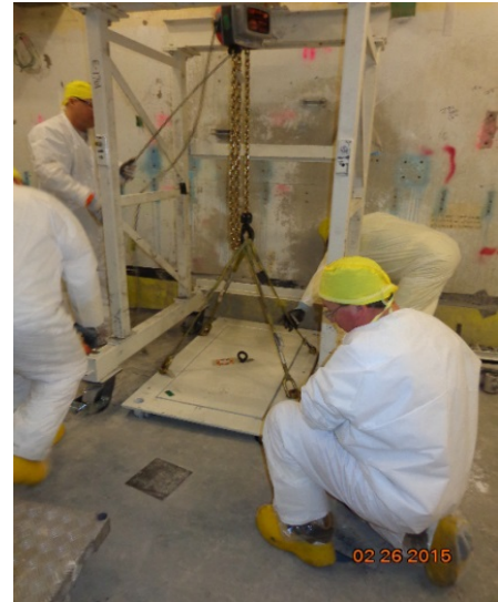
Figure 6. Workers install a ceiling hatch cover on a hatch opening.
