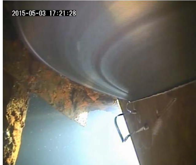
Fig. 13. Chute Cutting in PFSP
