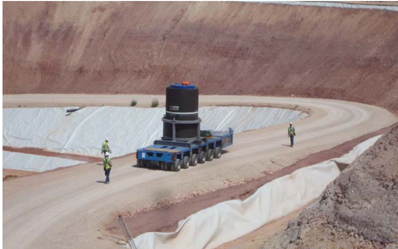
Fig. 2. Transporting a Modular Concrete Canister
