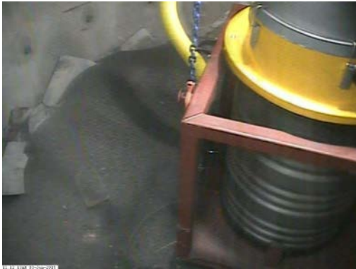
Figure 10: Suction unit at bottom
