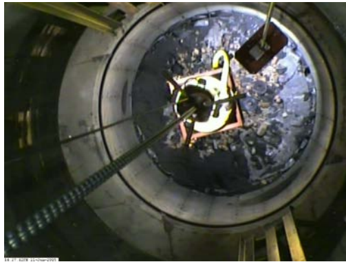
Figure 7: Complete suction unit and video unit in reactor shaft
