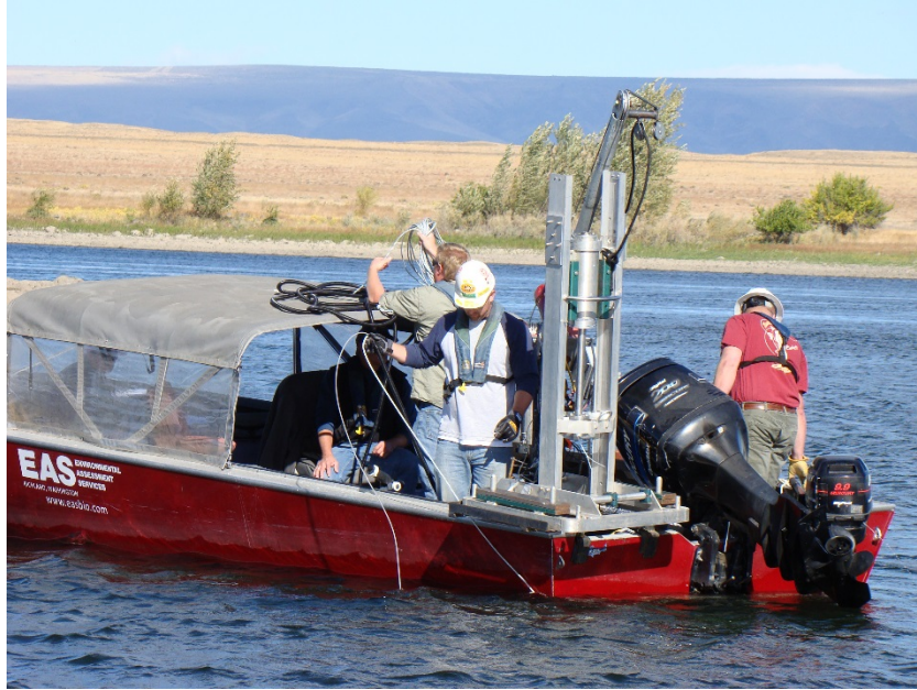
Fig. 3. Driving Frame Used to Install 100-BC Hyporheic Sampling Points
