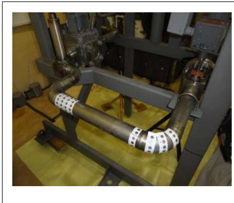
Fig. 3. UT Measurement Templates in Place on 51 mm (2 in.) Jumper Straight Section, 1.5D Elbow and < 1 Diameter Downstream of 1.5D Elbow in Preparation for Testing
