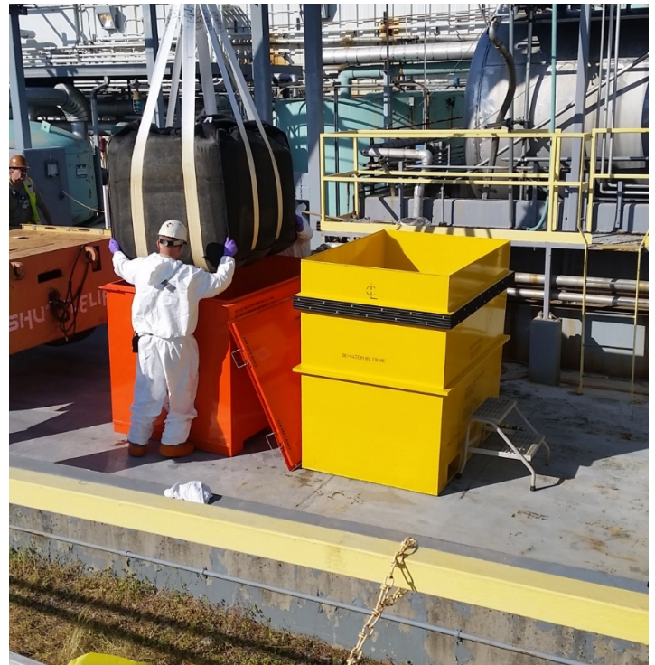
Figure 5 – Dewatering bag being lowered into the Shipping container
