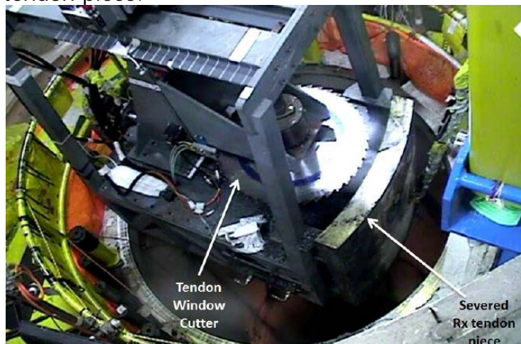
View inside of the reactor vessel and remote horizontal cutting tool. The specialty epoxy coated (white) surface minimized generation of airborne contamination. Shown below the Tendon Window Cutter removing a severed reactor tendon piece.
