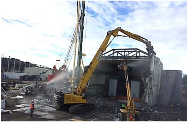
East end of the Refueling Building being demolished
