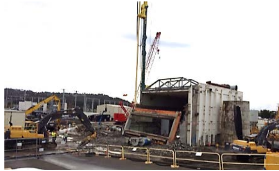
Pulling the 75 Ton bridge crane from the building
