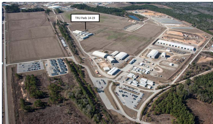
Figure 13 - E-Area Low Level Waste Storage Area and test location TRU Pad 17
