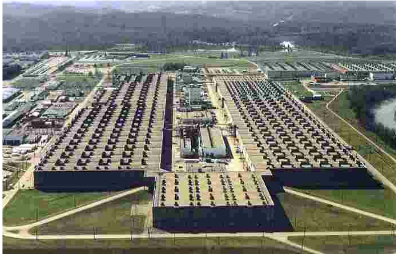
Figure 4A. The K-25 Building, Before D&D
