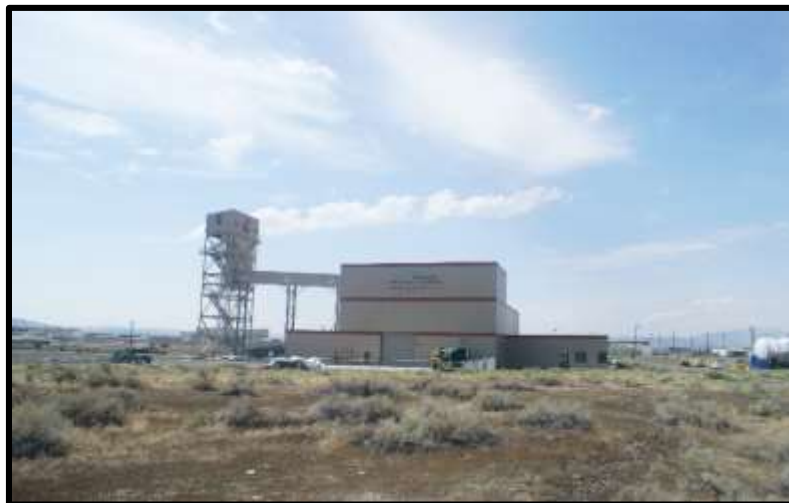
Figure 1. Energy Solutions Engineering Laboratory
