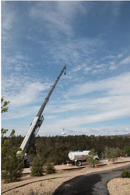
Figure 7. Hoisting from the excavation site and placement on flatbed for immediate delivery to the LANL waste staging area off public property.
