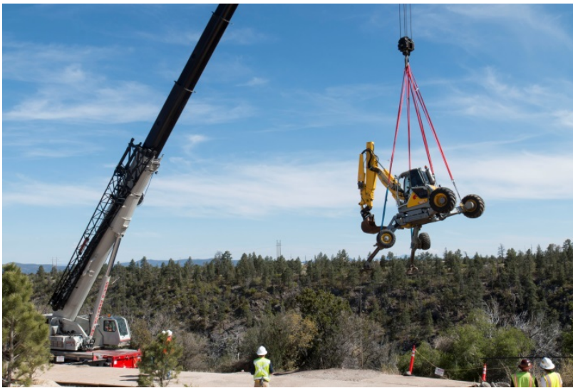
Figure 4. Photos of Linkbelt ATC 3275 lifting and lowering the Menzi Muck Spider Excavator to the excavation site. Photos courtesy of Los Alamos National Laboratory.
