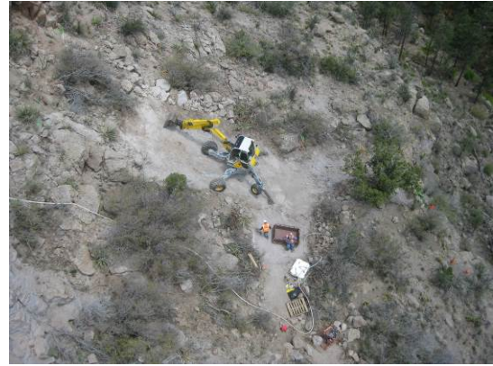
Figure 5. Menzi Muck 91-E spider excavator positioned on the SWMU 32-002(b2) excavation site.
