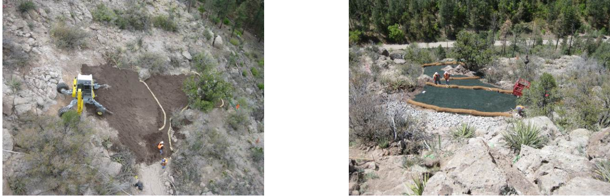
Figure 9. Site restoration at SWMU 32-002(b2) excavation site.
