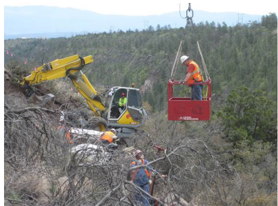
Figure 8. Hoisting personnel in man-basket at SWMU 32-002(b2) excavation site.
