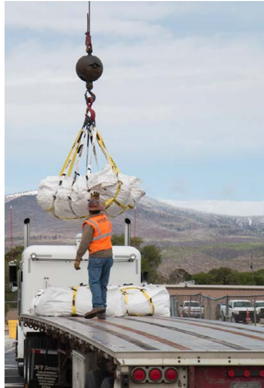
Figure 7. Hoisting from the excavation site and placement on flatbed for immediate delivery to the LANL waste staging area off public property.
