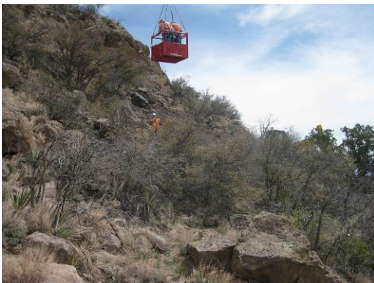
Figure 8. Hoisting personnel in man-basket at SWMU 32-002(b2) excavation site.
