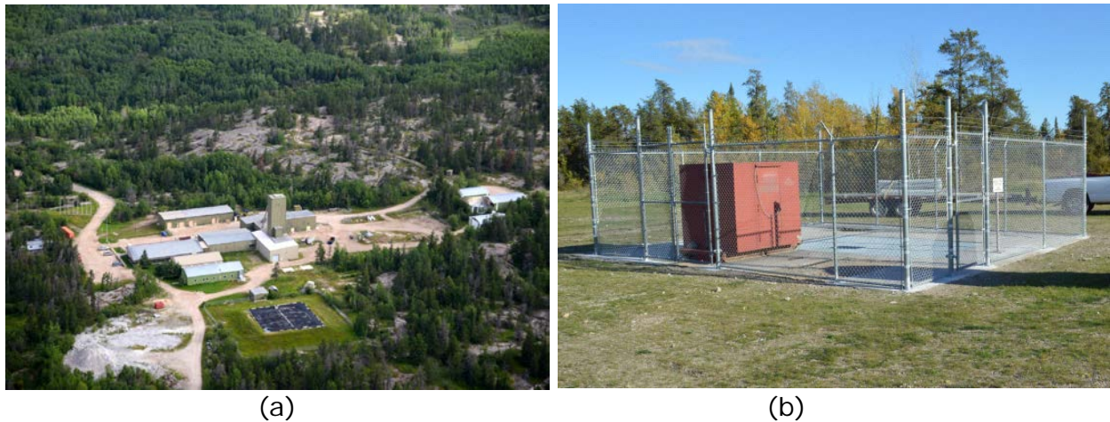
Fig. 4. (a) Original URL facility layout. (b) ESP monitoring enclosure in October 2015
