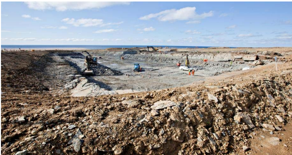
June 2012 – excavation work
