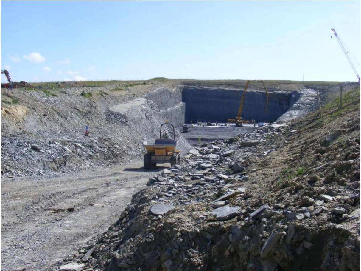
August 2012 – installation of floor slab
