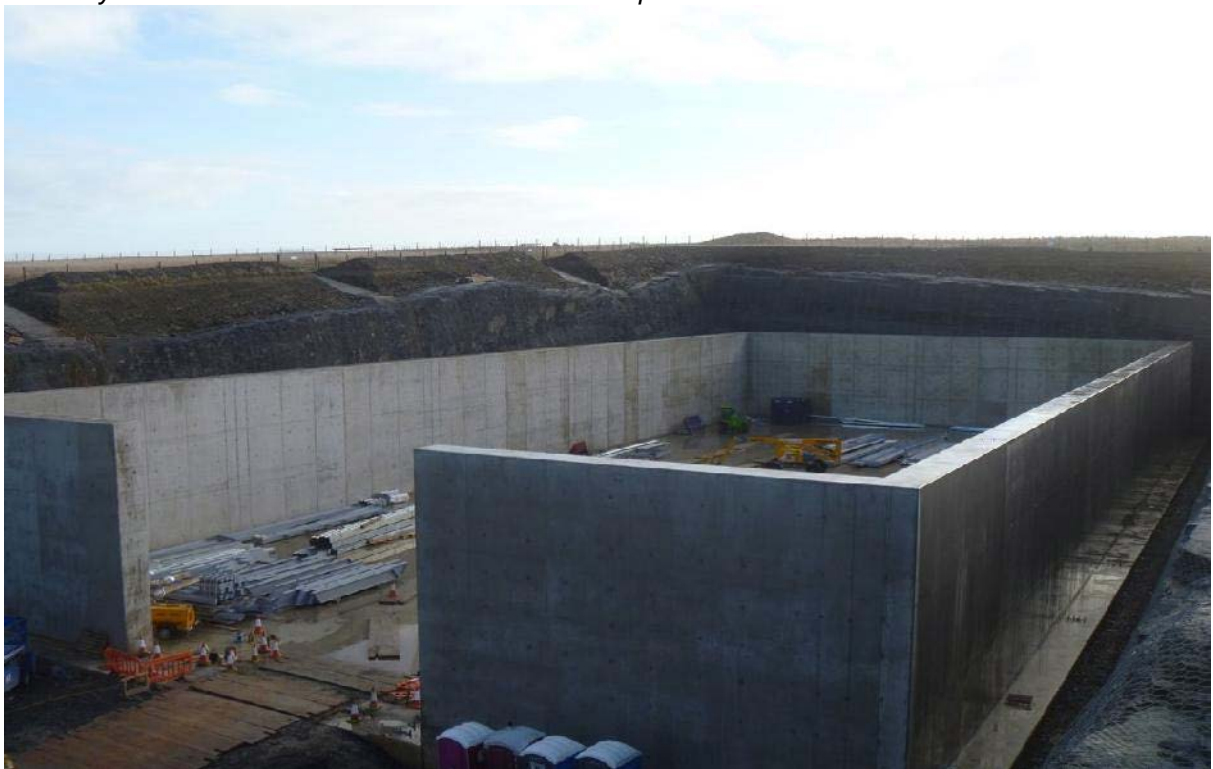
February 2013 – construction of re-inforced walls complete
