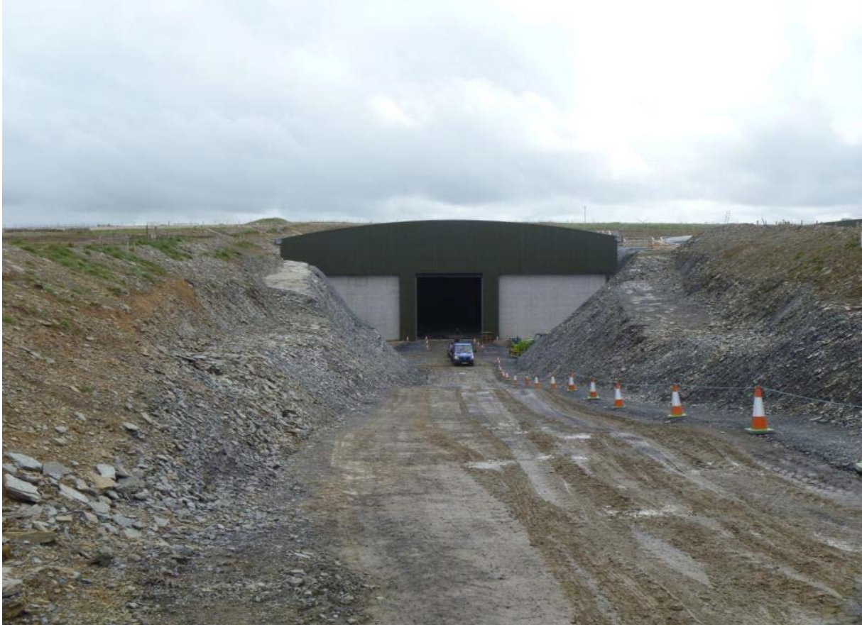
May 2013 – roof installation complete
