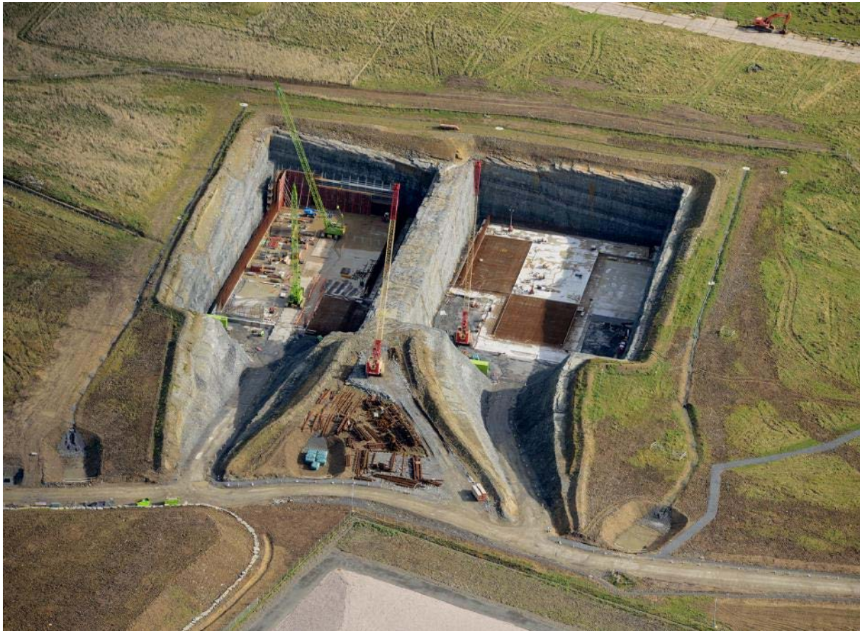
October 2012 – aerial view of construction
