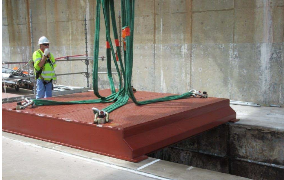
Fig. 8 Modular Shielding System (horizontal plug, FWH example)
