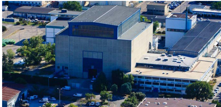
Fig. 1. View of the G1 Reactor Building.
