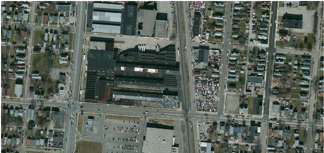
Figure 2: Aerial view of the Hamilton, Ohio, site prior to demolition of the building
