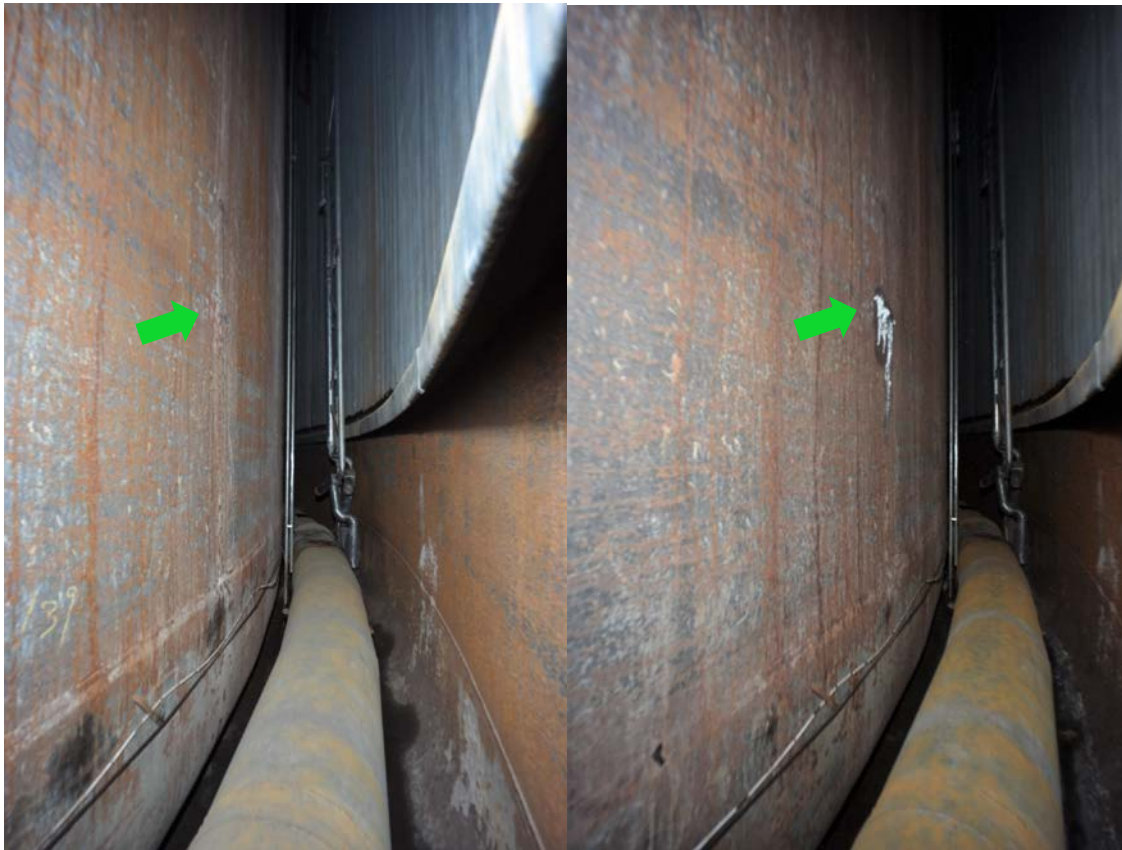
Figure 2. Known Leak Site Before and After Liquid Additions
