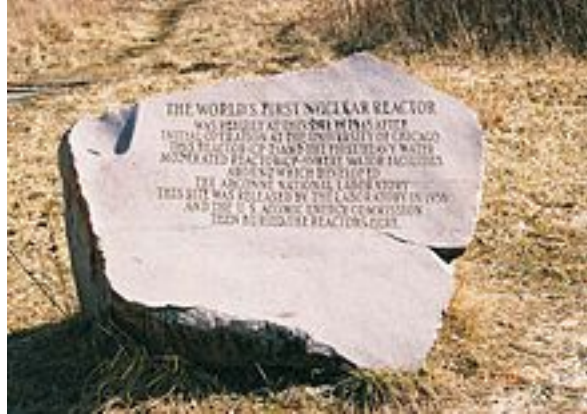
Figure 3. Plot M marker at the Forest Preserve District of Cook County. Obvious weathering has occurred on the monument enhancing a natural fracture in the stone that is beginning to intersect with the inscription.
