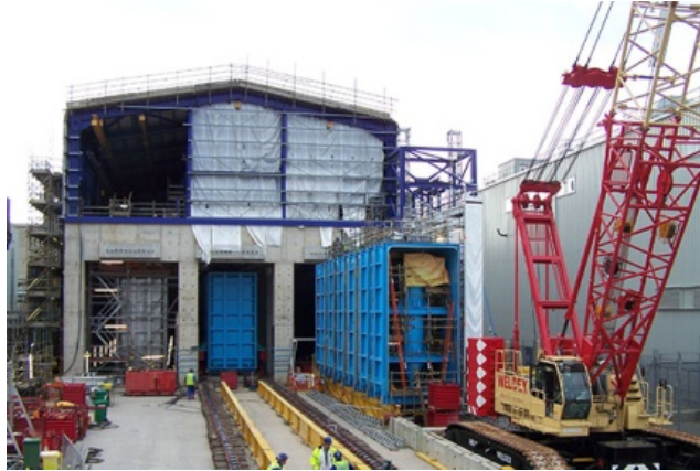
Fig. 1. SPP1 Sludge Settling Tanks
