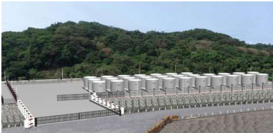
Fig. 2. Schematic depiction of ISFSI Dry-Storage Facility at Chinshan
