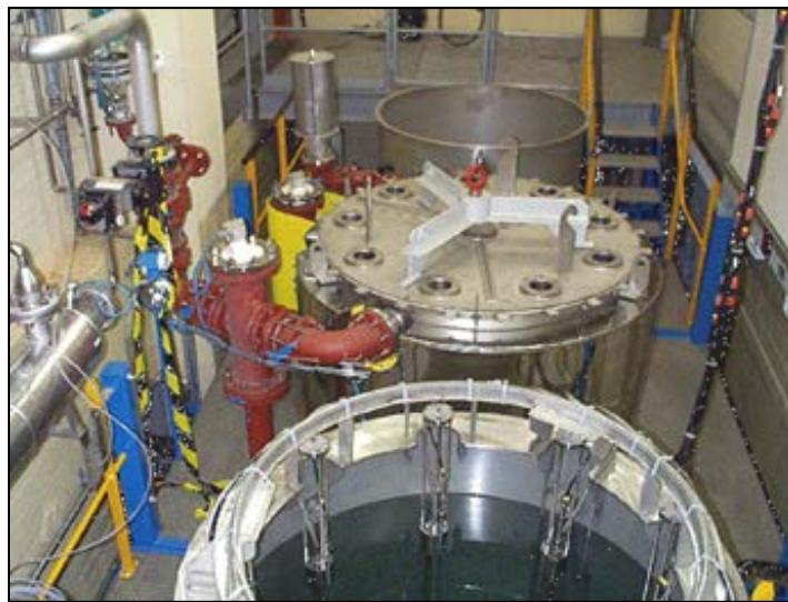
Figure 11: MEDOC® chemical decontamination workshop
