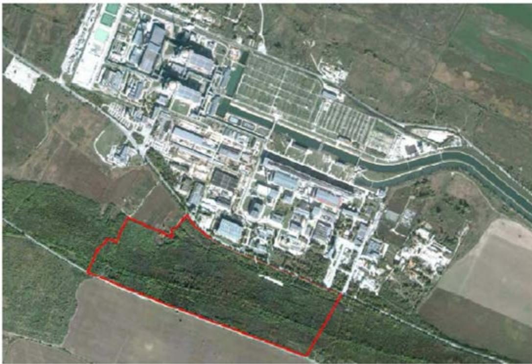
Figure 1: Radiana Site where the NDF will be constructed in relationship to the KNPP
