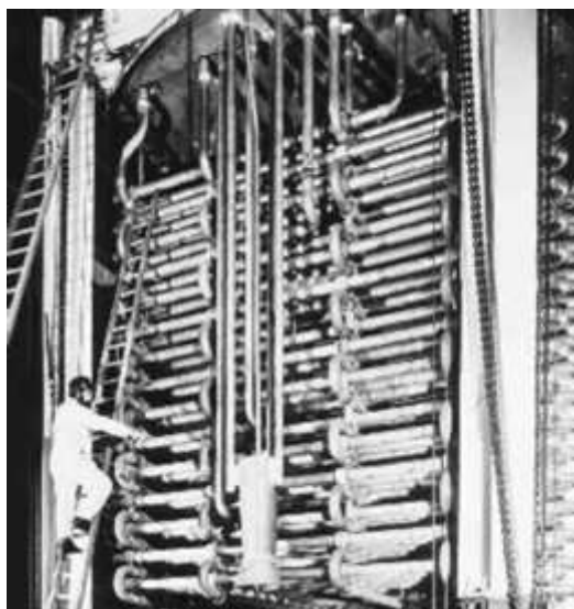
Fig. 4. New-side HAST during construction
