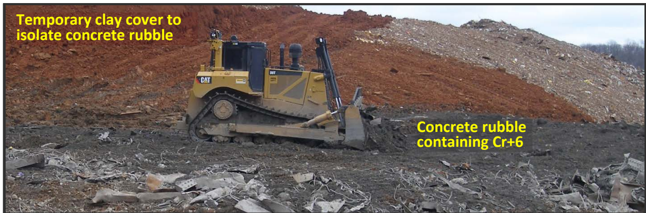
Fig. 2. Placement of Pulverized Concrete Rubble from K-33.
