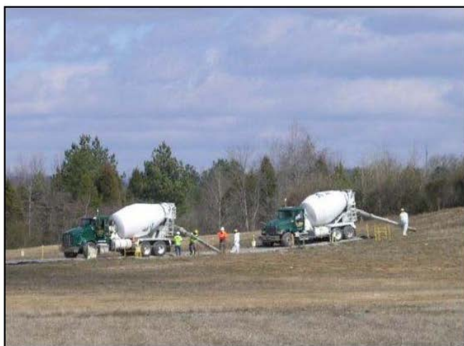
Fig. 4. Grouting duct row (left) and concrete-filled vault adjacent to creek (right). Photo: DOE
