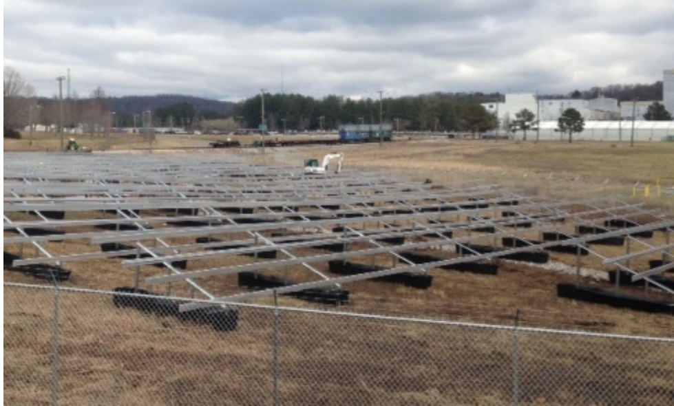
Fig. 6. Powerhouse Six racking system sitting on the GameChange® Pour-in-Place™ ballasted system. Photo: RSI
