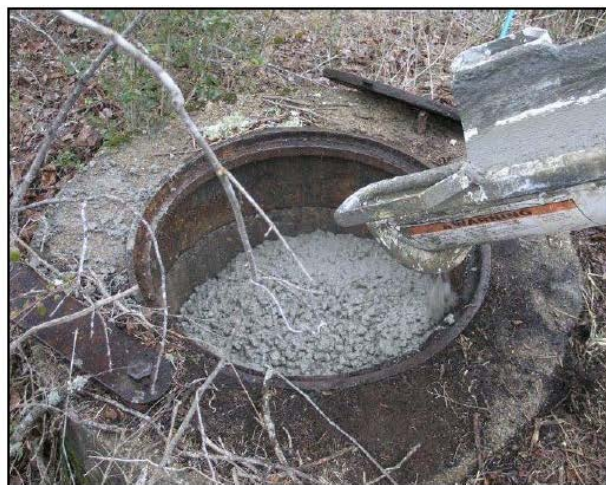
Fig. 4. Grouting duct row (left) and concrete-filled vault adjacent to creek (right). Photo: DOE
