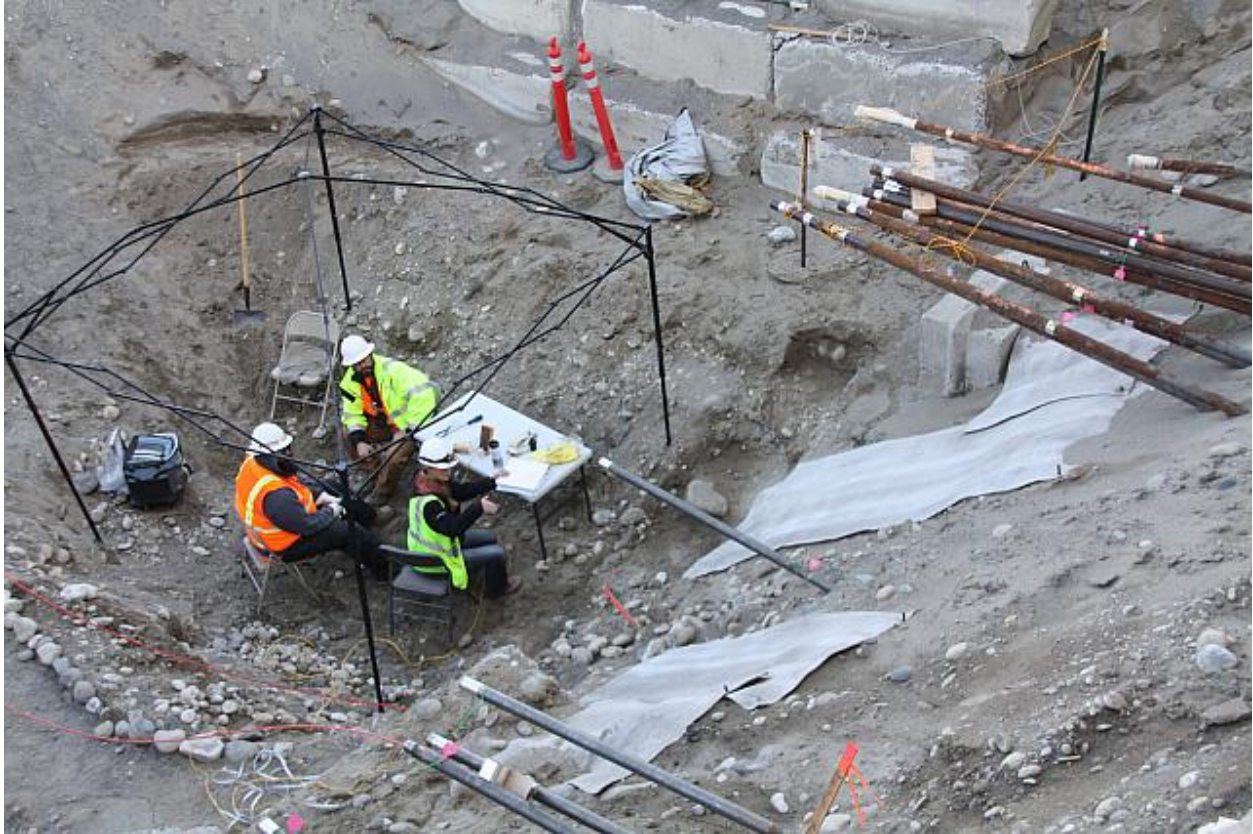
Fig. 8. Geoprobe Tubes Placed for Investigation of West Side of 324 Building B-Cell, October 2014.
