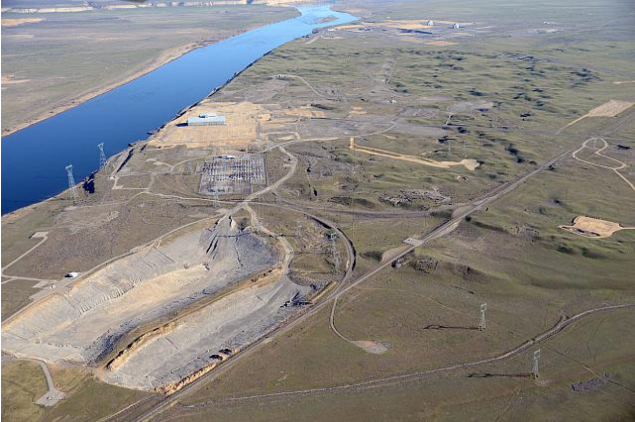
Fig. 4. Cleanup and Revegetation at the 100-N Area, March 2015.
