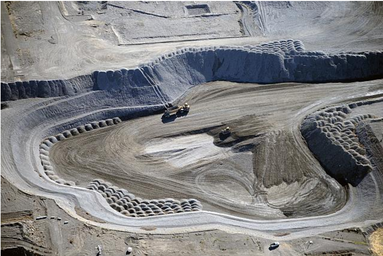
Fig. 3. Backfill Activities at the 100-D-100 Chromium Contamination Waste Site, March 2015.
