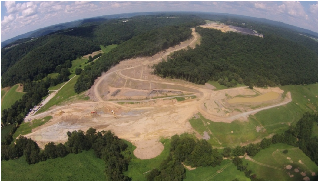
Fig. 4. Ridge Haul Road.
